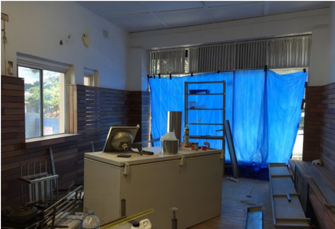
Figure 43 | Interior of the retail area of No. 443-445 in 2015. There is no evidence of Inter-war fabric left apart from the battened ceiling, which was retained.
