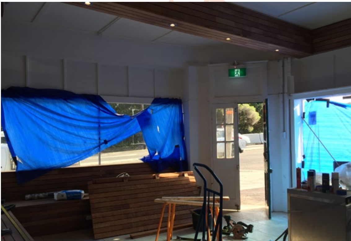
Figure 44 | Interior view of the entrance in 2015. The double doors and the shopfront hamper panels are the only original fabric left; they were retained.
